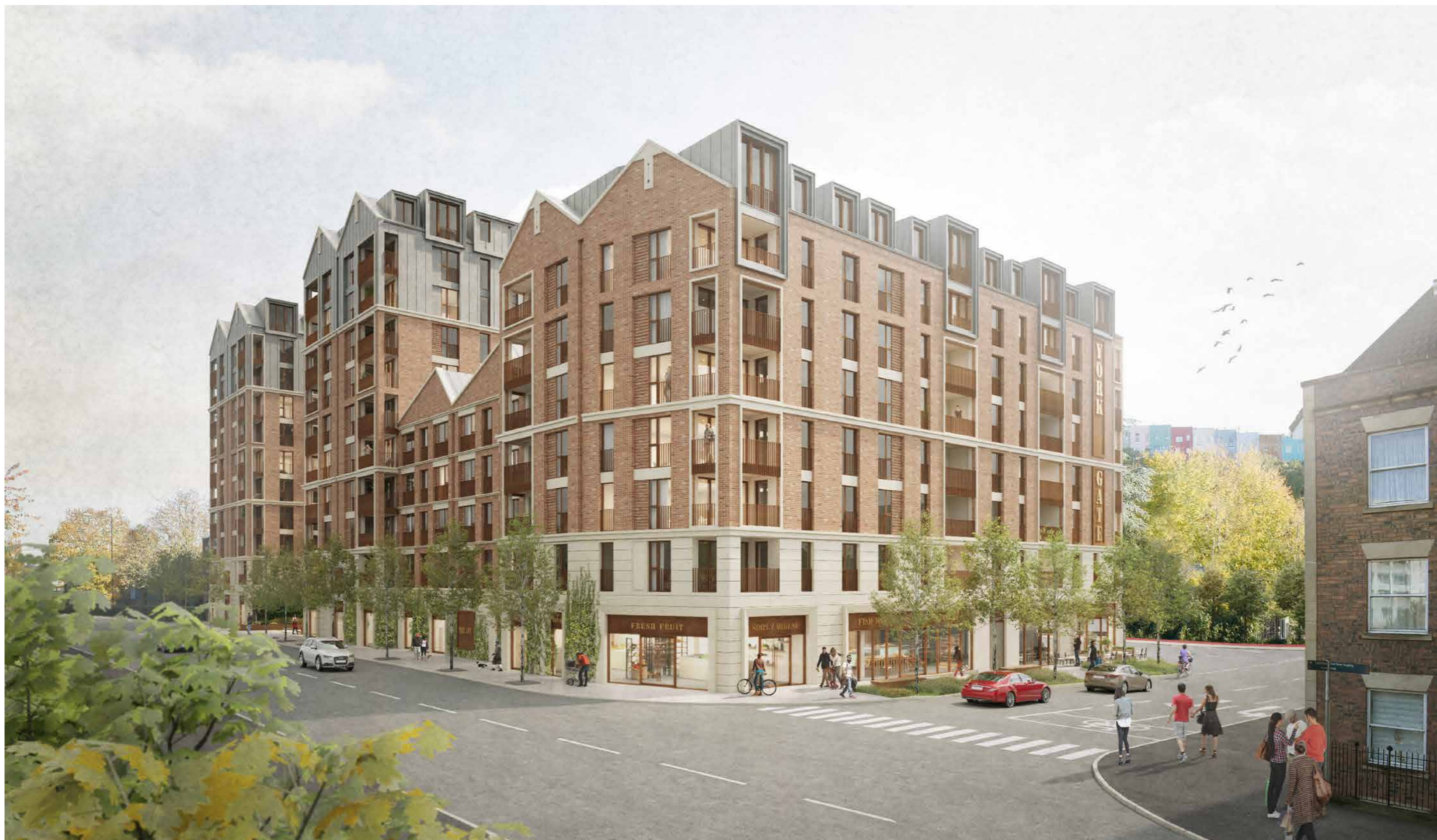
Submitted rendered view at junction of York Road and St Luke's Road
